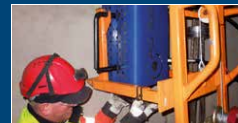
Multi-strand stressing jacks Bündelspannpresse
